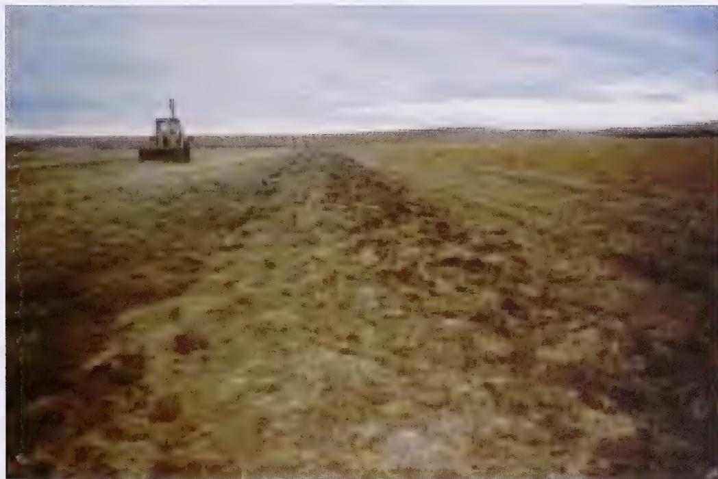
Photo 33 Topsoil and sod is replaced keeping the sod as intact as possible. Sod was stripped and replaced within 48 hours.
